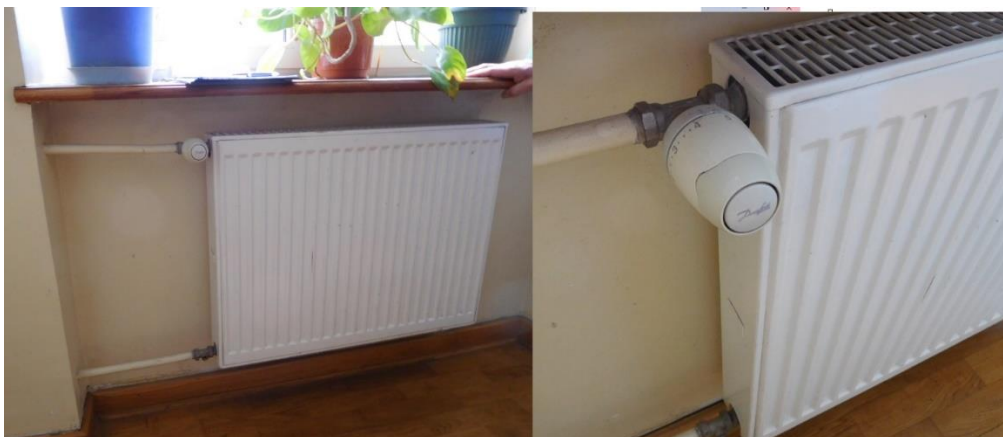
Figure 72 Water convectors with thermostatic valves
