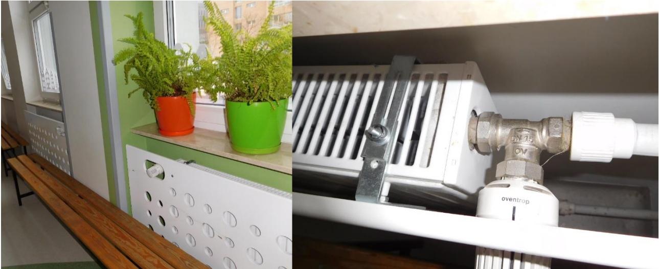
Figure 41 Water convectors with thermostatic valves
