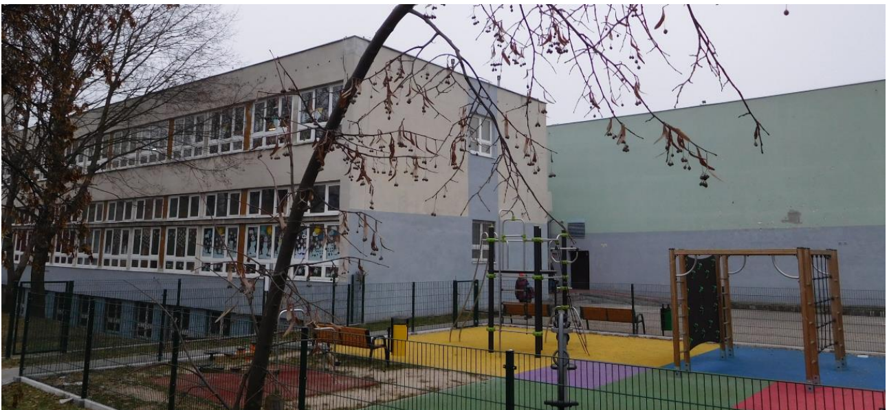
Figure 27 South-west side of the building
