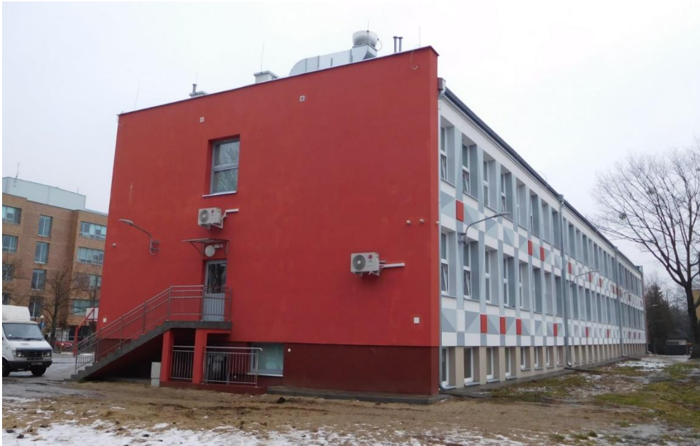
Figure 43 South-west side of the building
