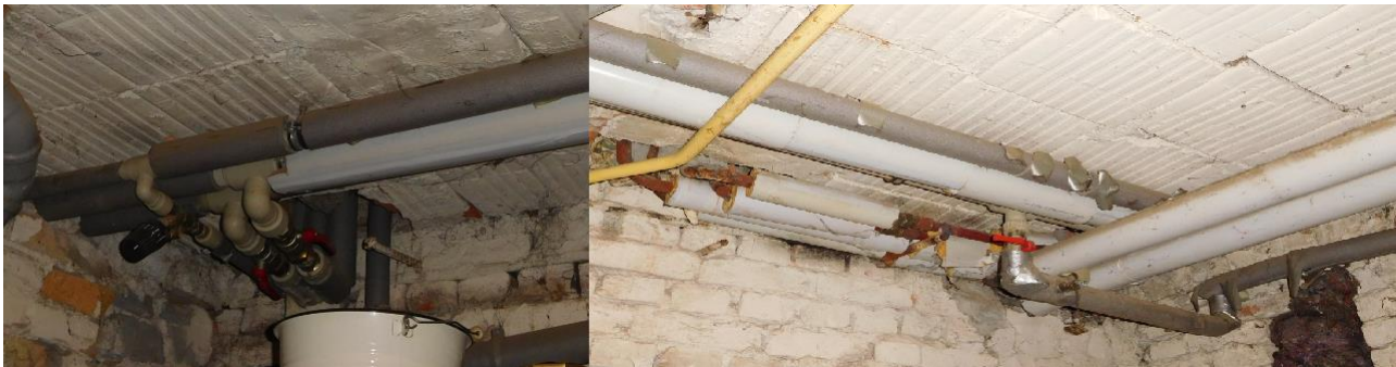
Figure 3 Insulated pipes
