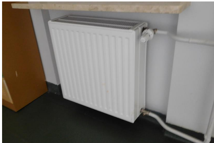
Figure 4 Water convectors with thermostatic valves
