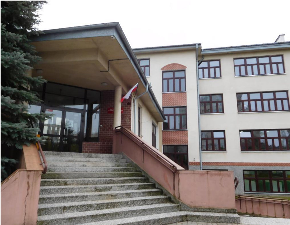
Figure 19 Main entrance (north elevation)
