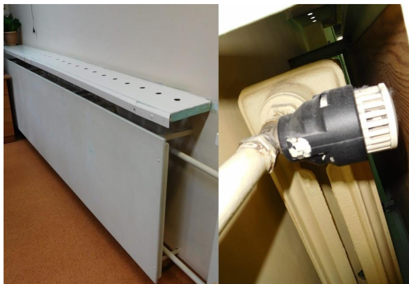
Figure 35 Water convectors with thermostatic valves
