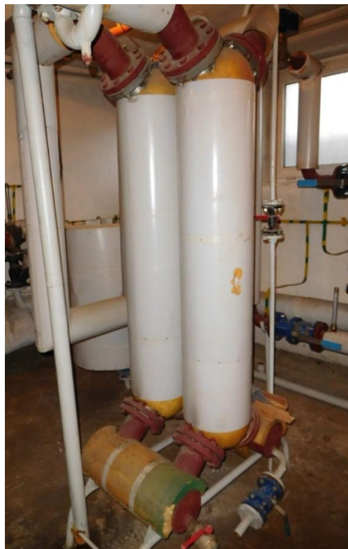
Figure 59 Heating source in the building
