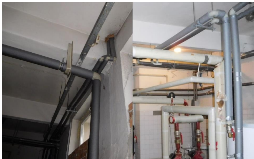
Figure 40 Insulated pipes
