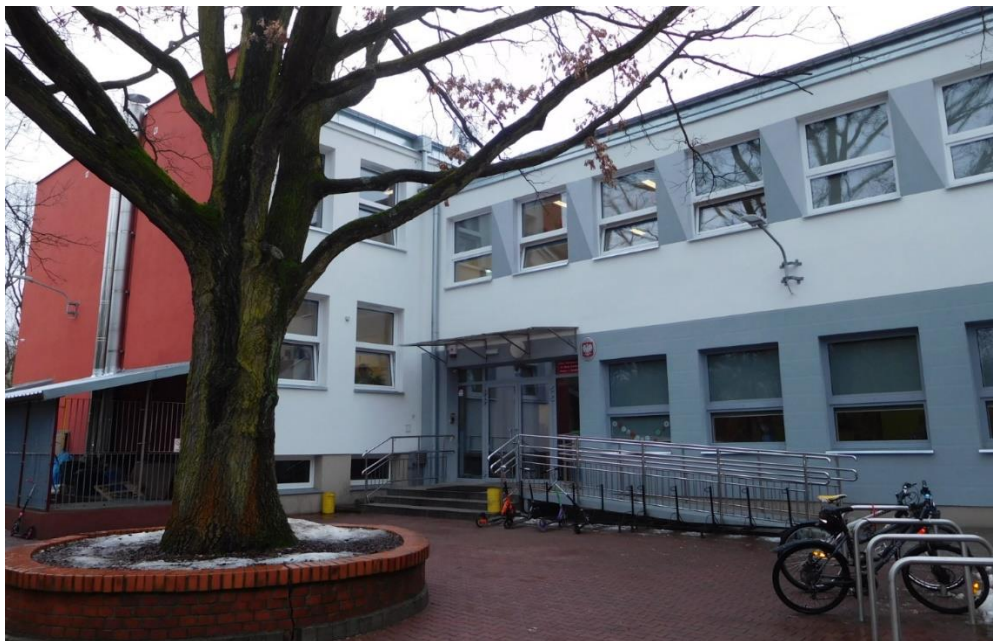
Figure 44 North-east side of the building
