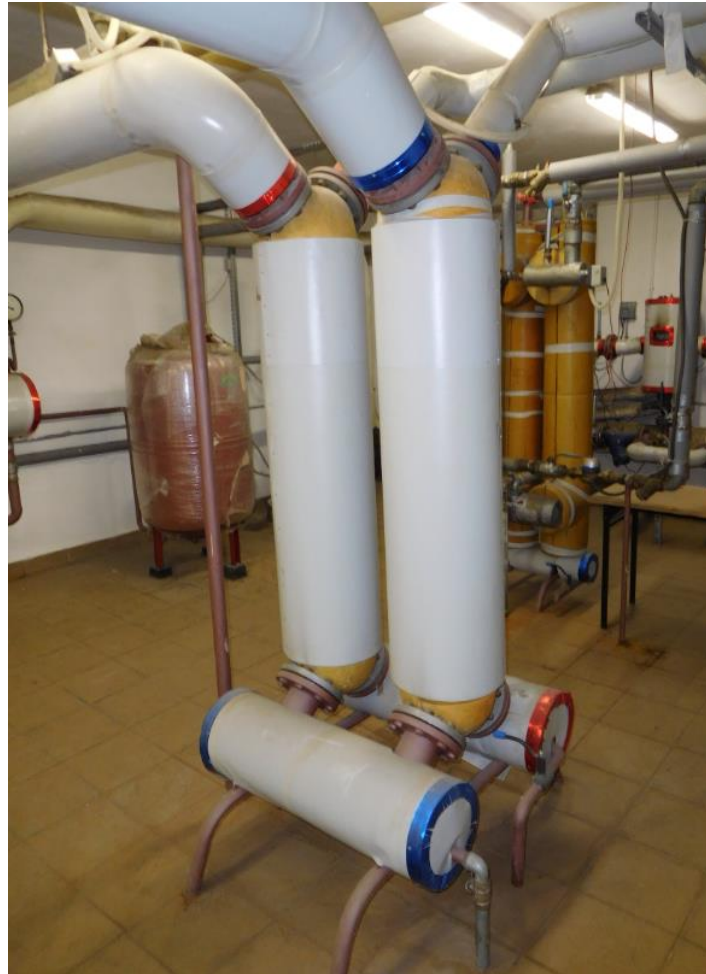
Figure 22 Heating source in the building
