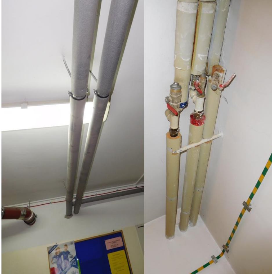
Figure 71 Insulated pipes
