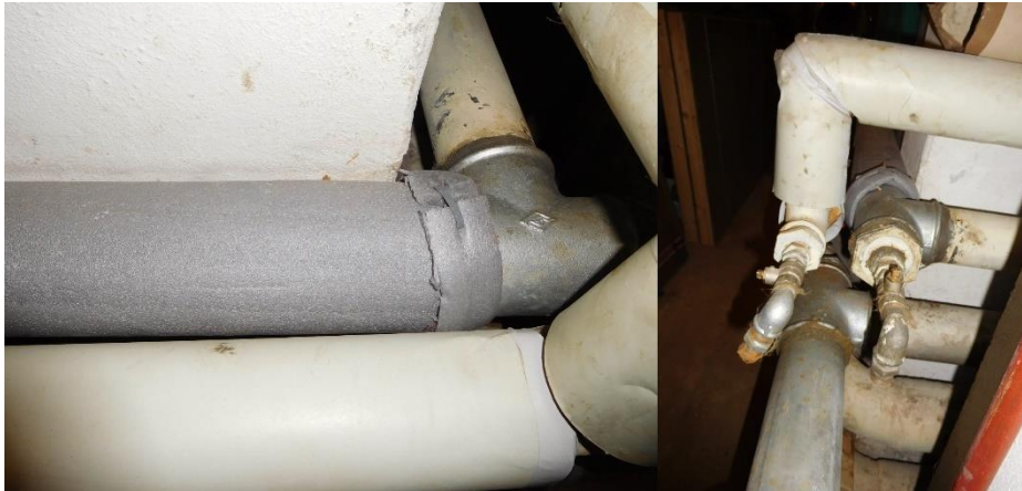
Figure 34 Insulated pipes
