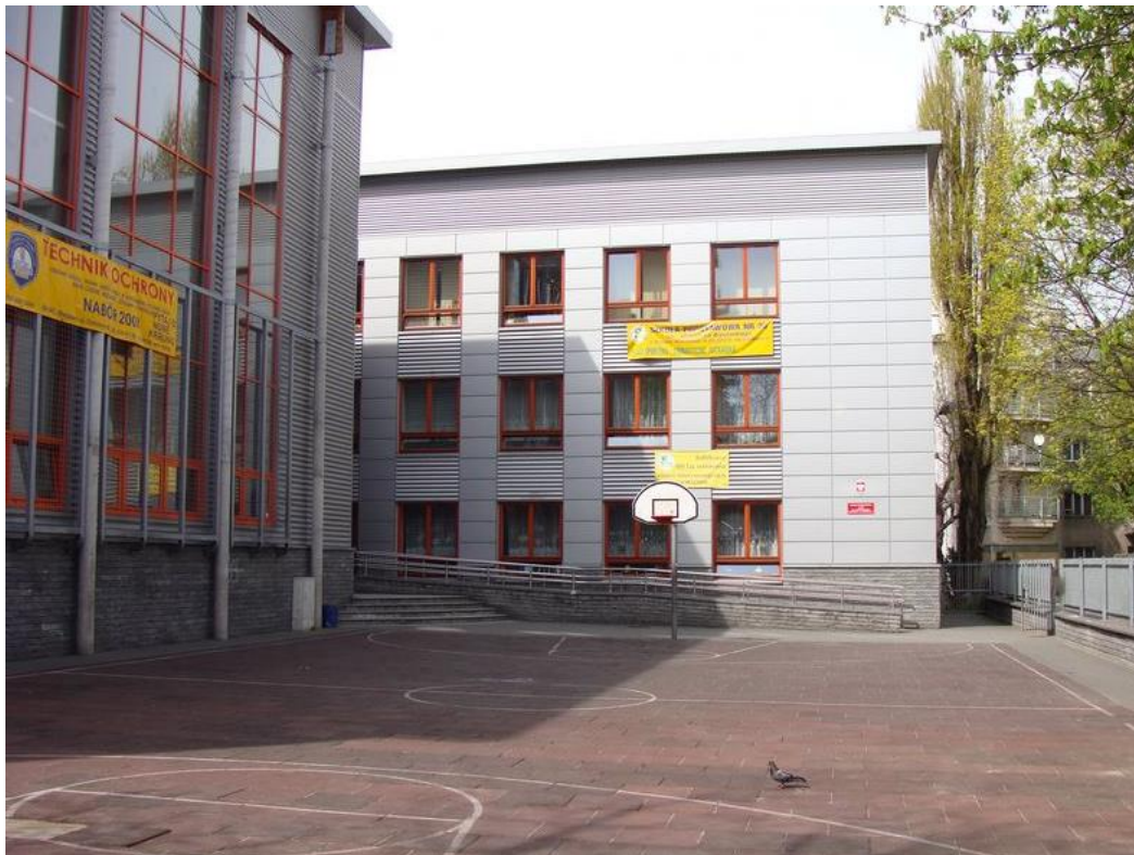
Figure 75 North-western side of the building
