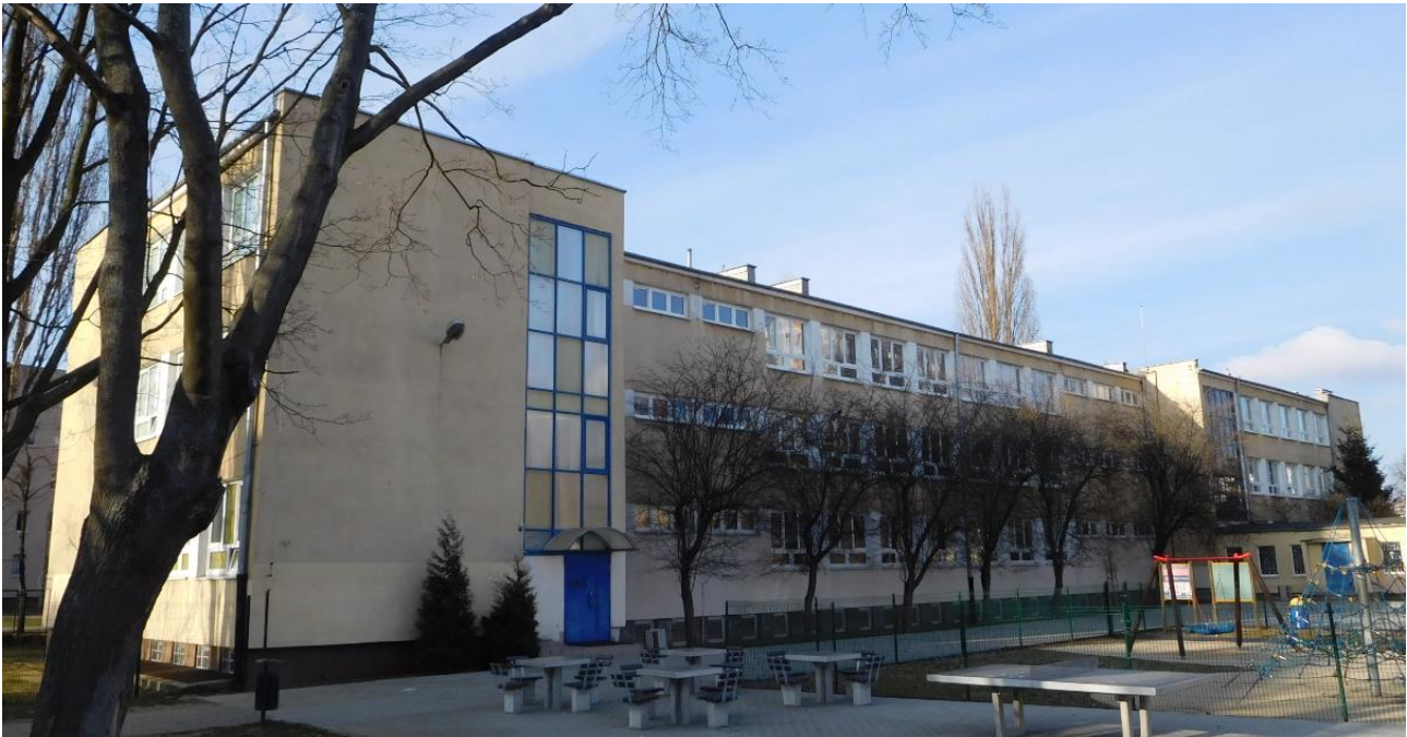
Figure 63 South-east side of the building
