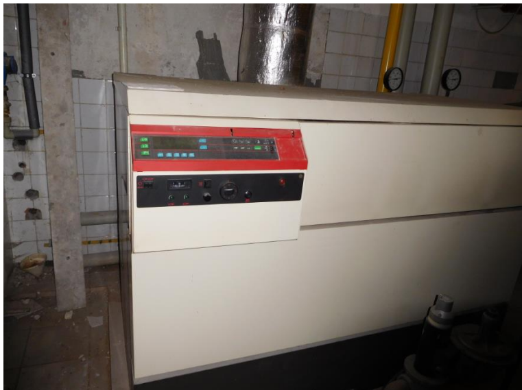
Figure 39 Heating source in the building
