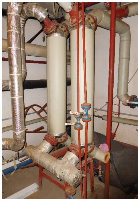
Figure 49 Heating source in the building
