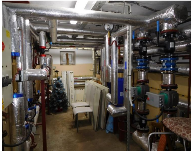
Figure 2 Heating source in the building
