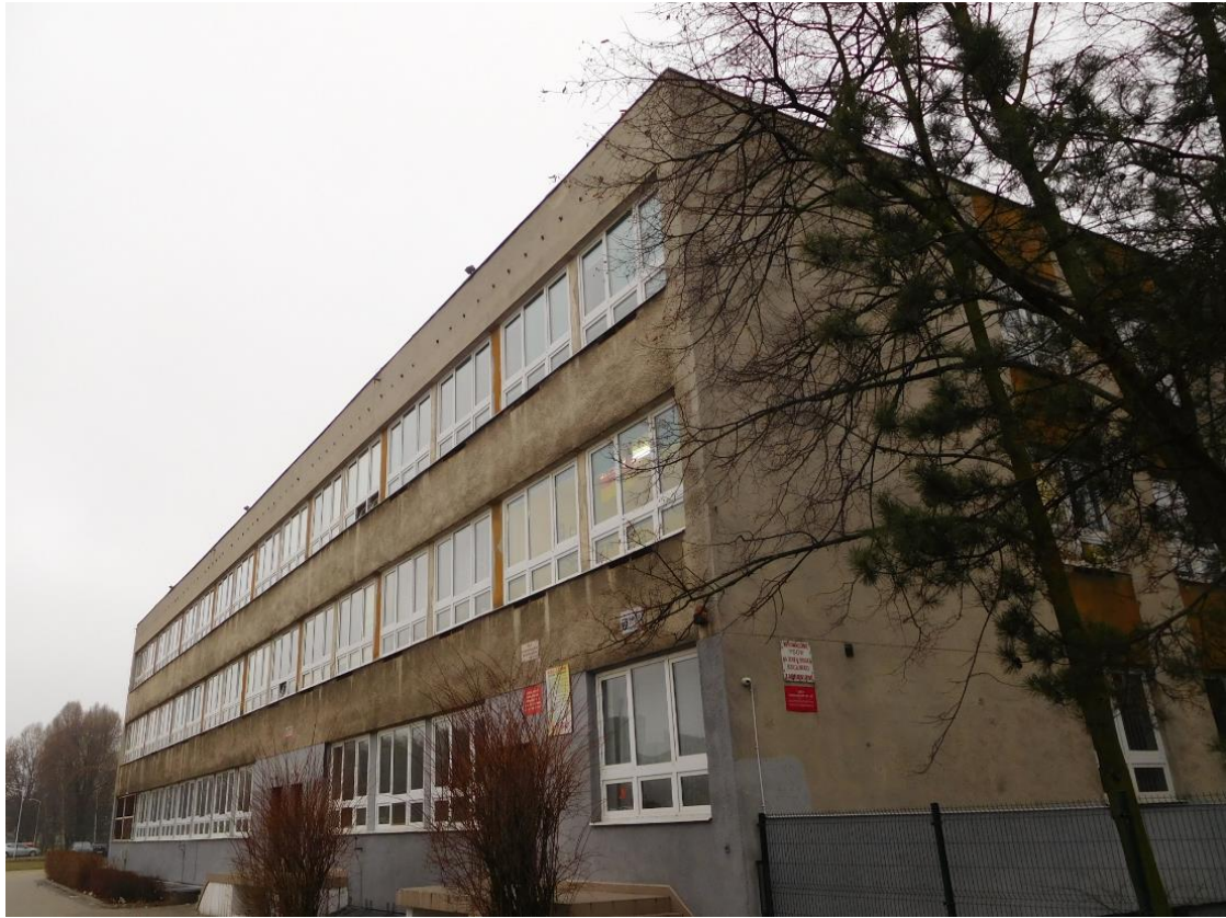
Figure 26 East side of the building
