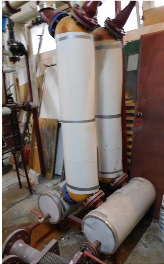
Figure 14 Heating source in the building
