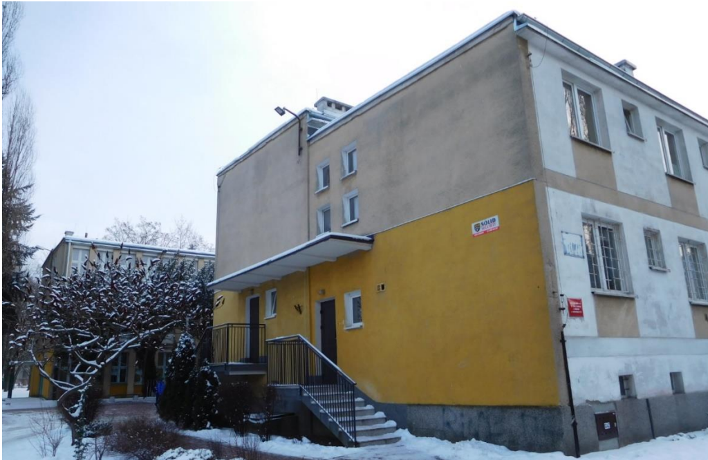
Figure 54 North-west side of the building
