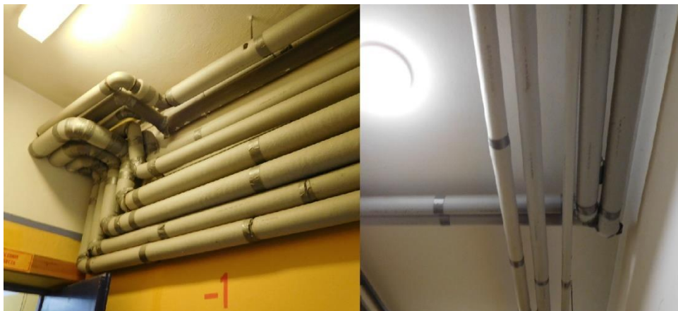
Figure 15 Insulated pipes
