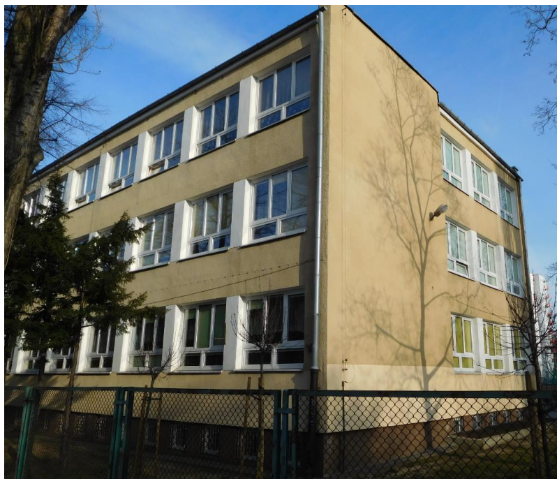
Figure 64 South-west side of the building
