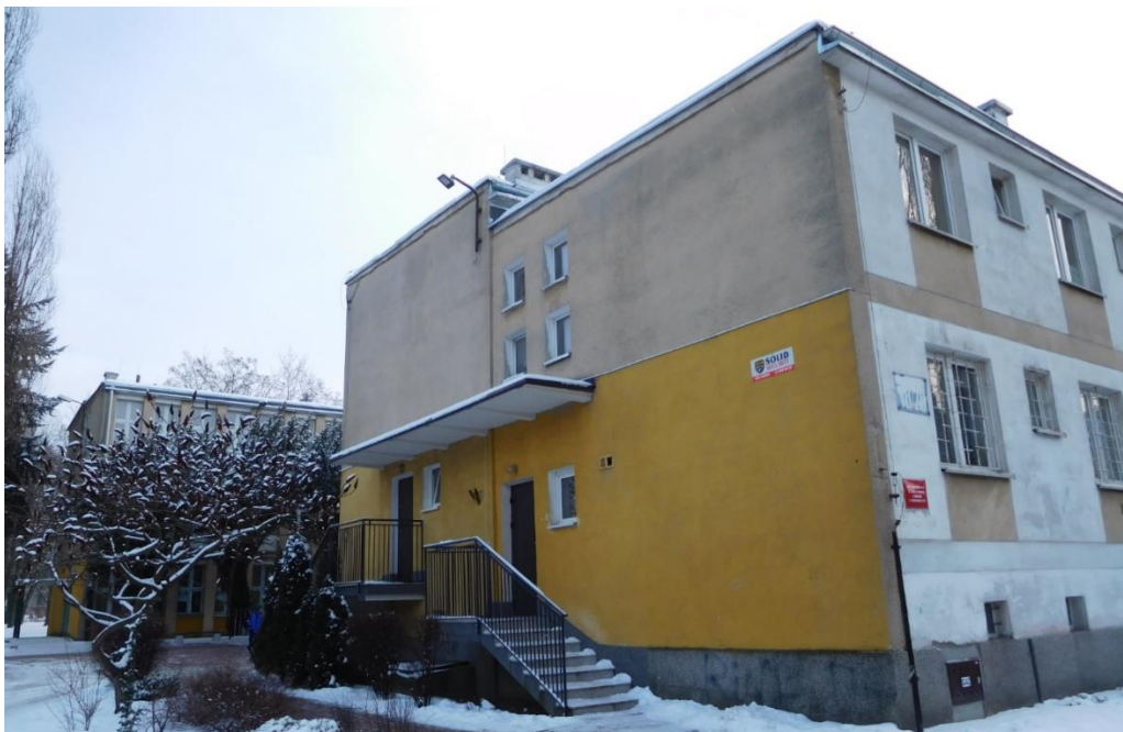
Figure 60 North-western side of the building
