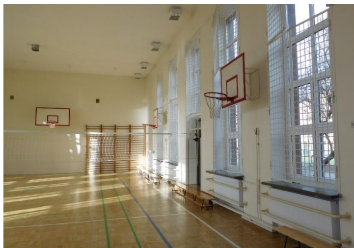
Figure 7 Sport hall ventilation
