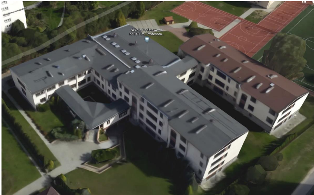
Figure 22 School SP 340 building (source: Google Maps)
