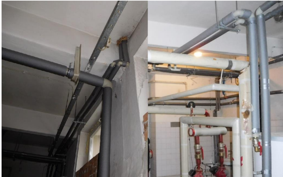
Figure 44 Insulated pipes
