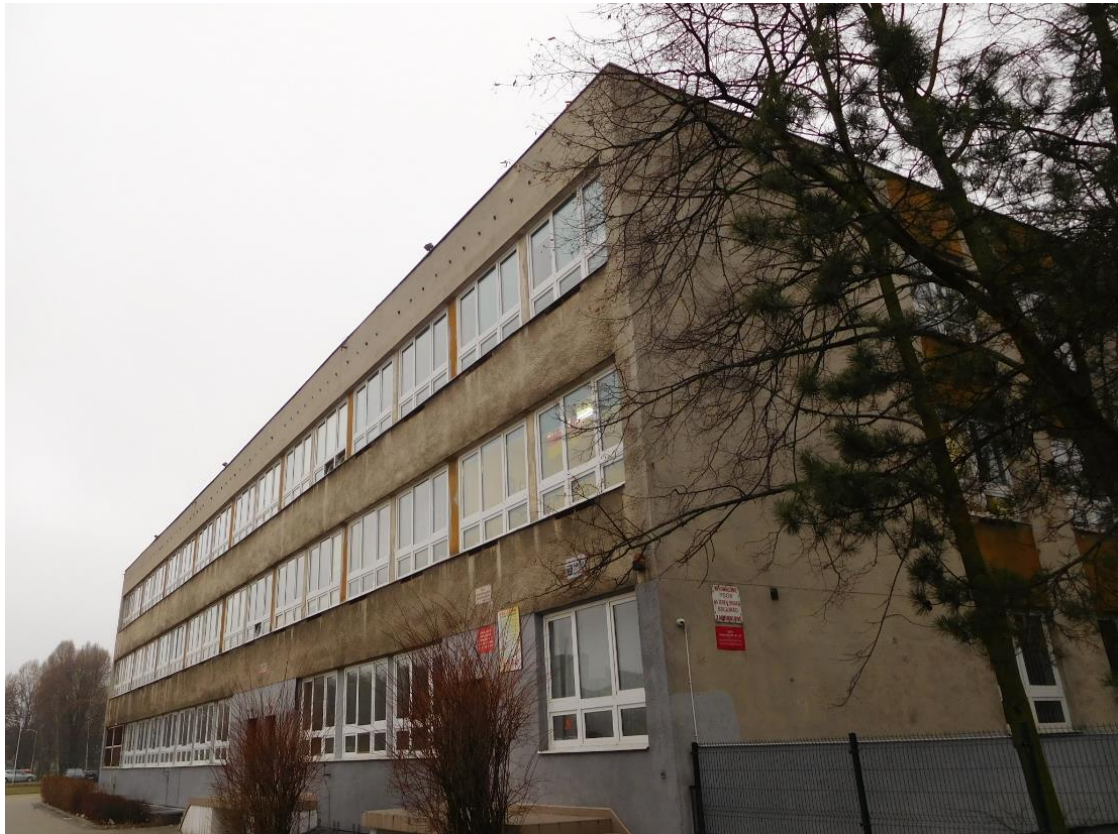
Figure 30 East side of the building
