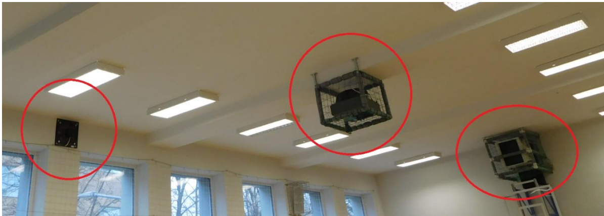
Figure 47 HVAC installation in the sport hall
