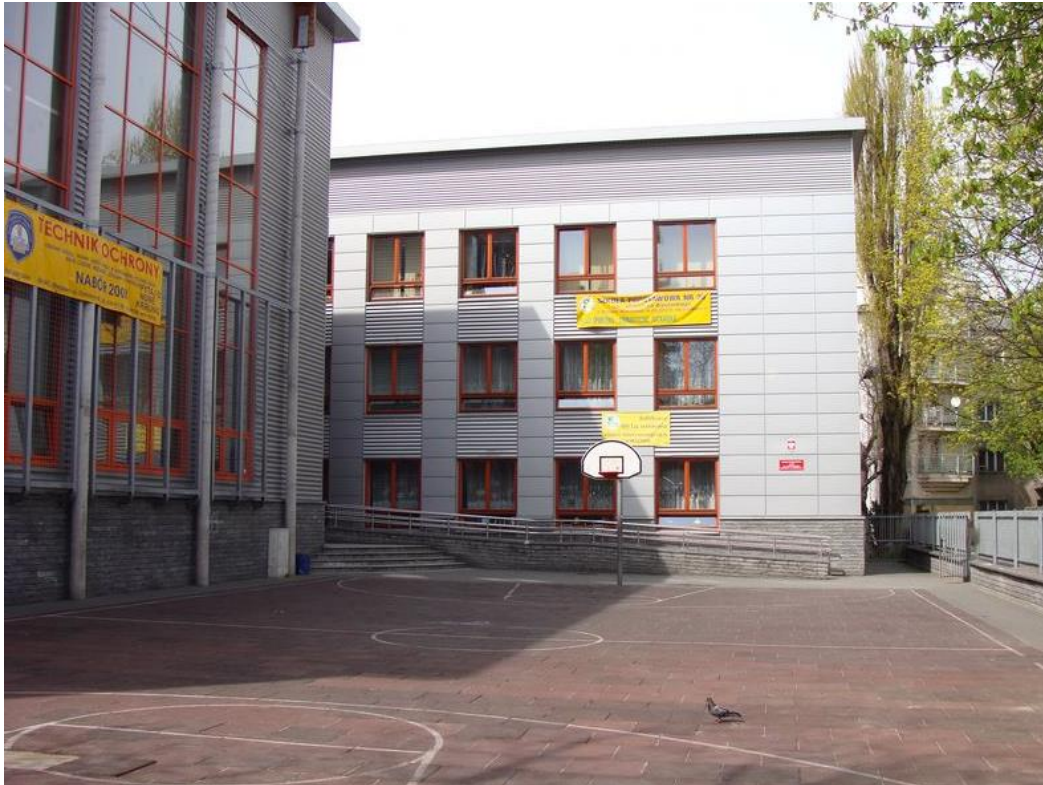
Figure 83 North-western side of the building
