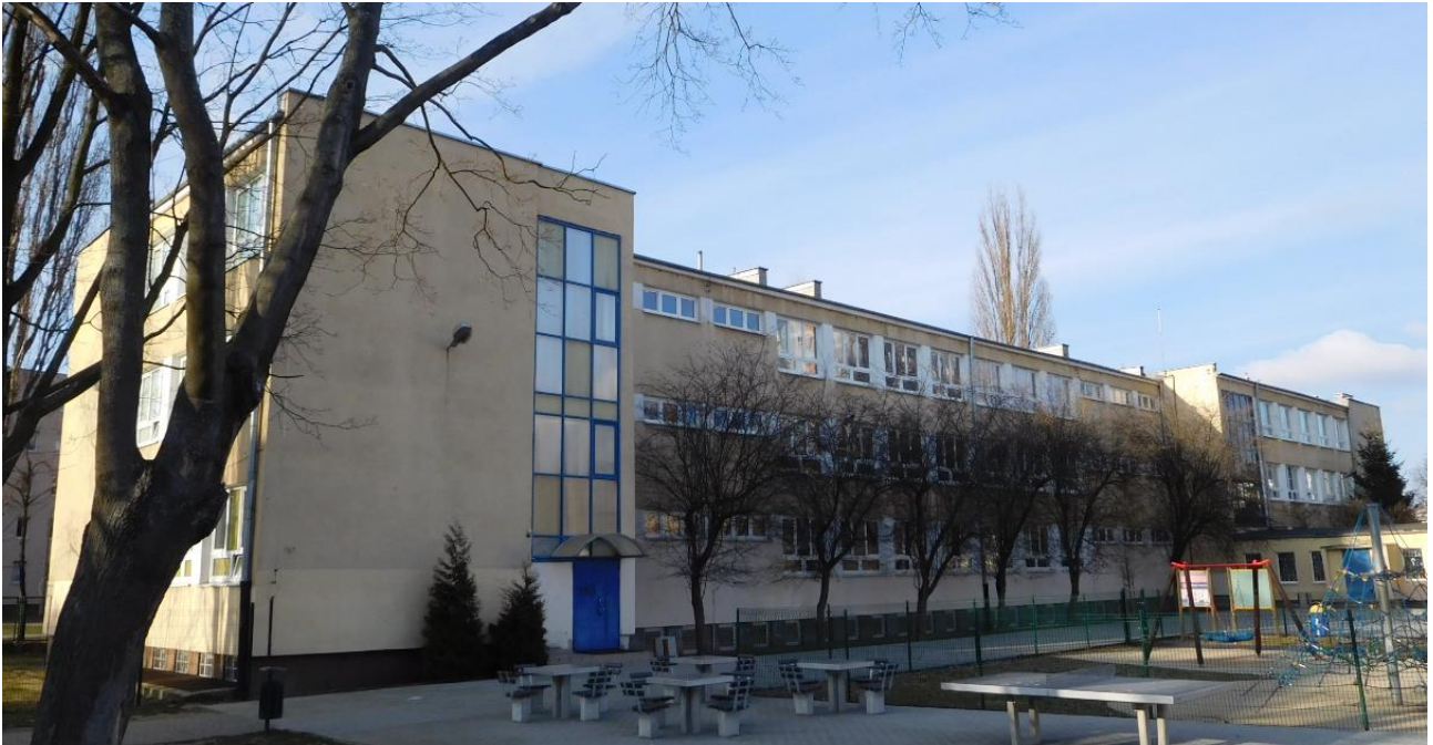
Figure 70 South-east side of the building
