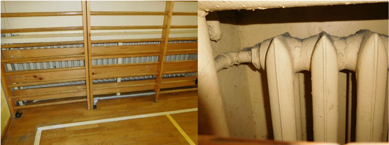
Figure 68 Iron ribbed convectors in the sport hall
